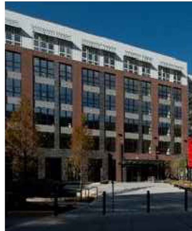
Masonry Fenestration and Brick Articulation
